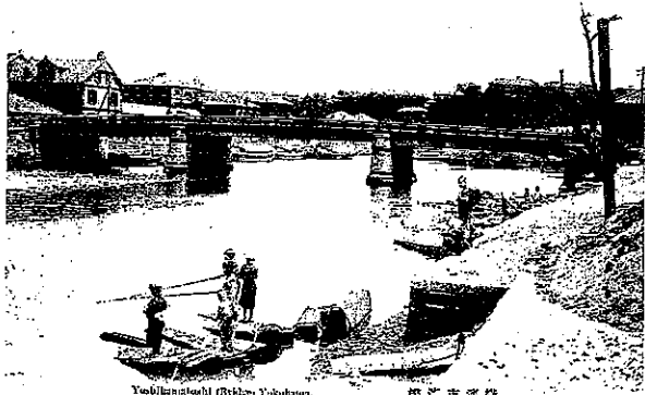
Yoshida Bridge (Rikkyo, Yokohama) 橋田吉濱橋
